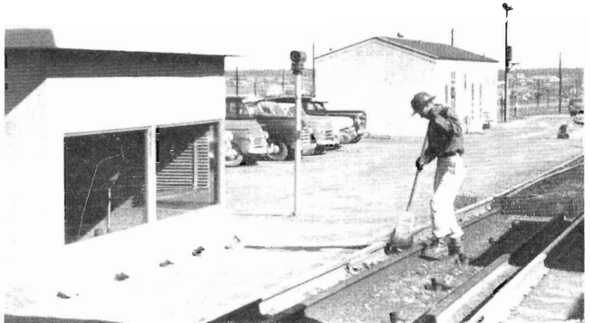
Train examiners' pit cabin for undergear inspection. Note the lights at ground level for night operation.
