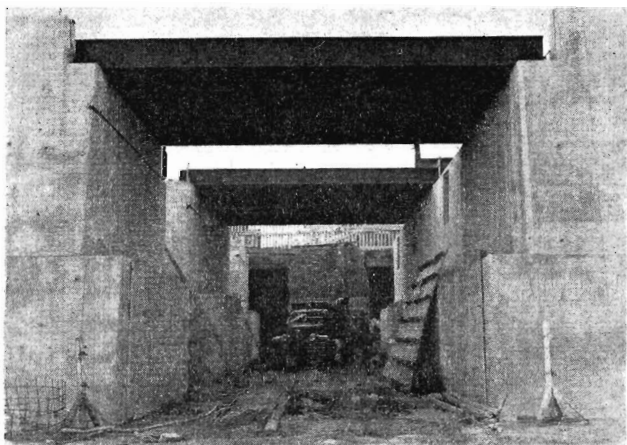
Ramp from main subway under construction and, below, the main subway. Floor level of the subway can be seen by the concrete projection about half-way up the walls.
