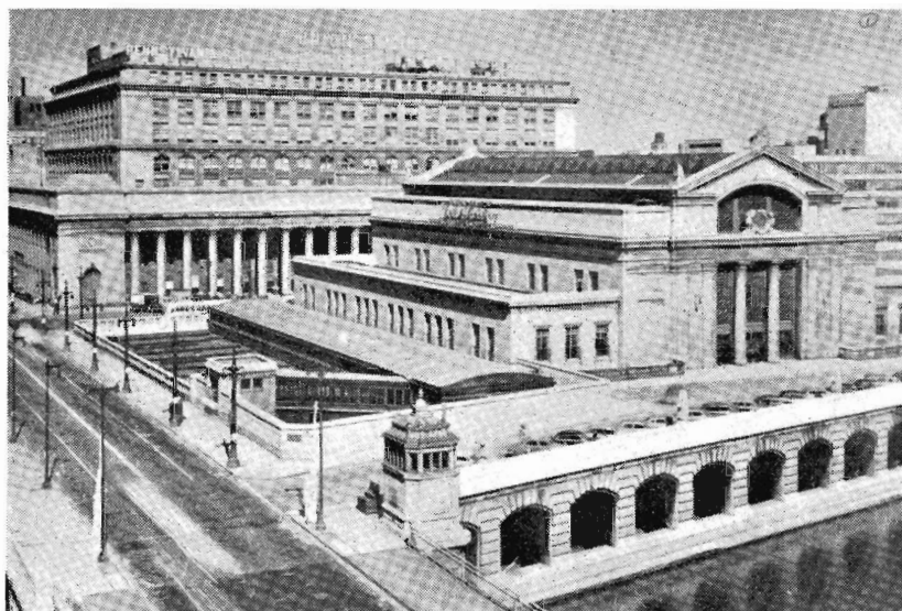
Union Station, Chicago's most important passenger terminal.
