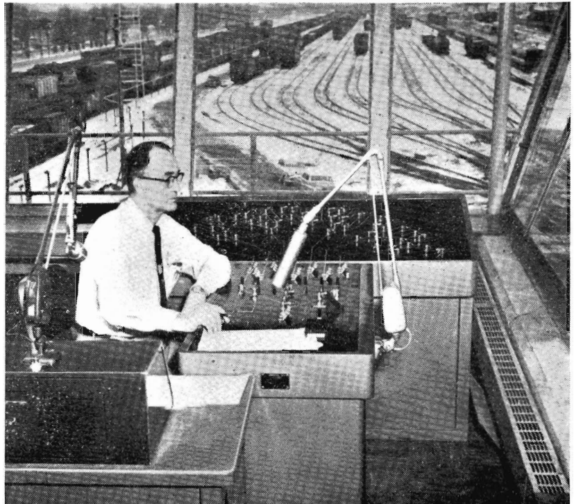
Retarder operator in control tower can exercise manual control of retarders and points if necessary.
