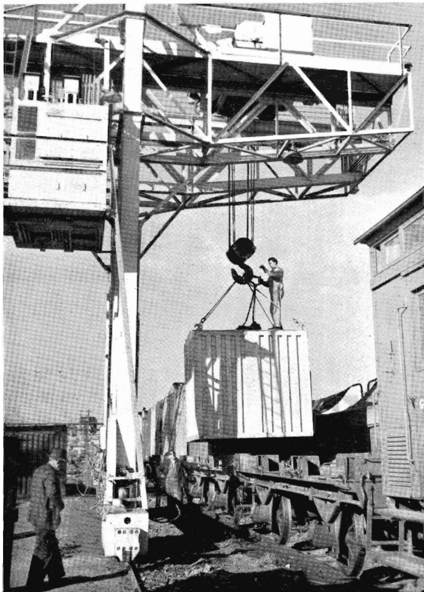
Loading steel freight container onto specially fitted flat truck.
