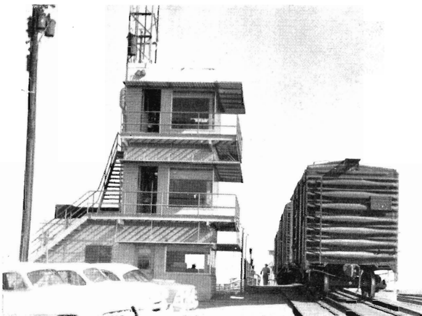
Control tower and "hump" at Englewood Yard, near Houston, Texas.
