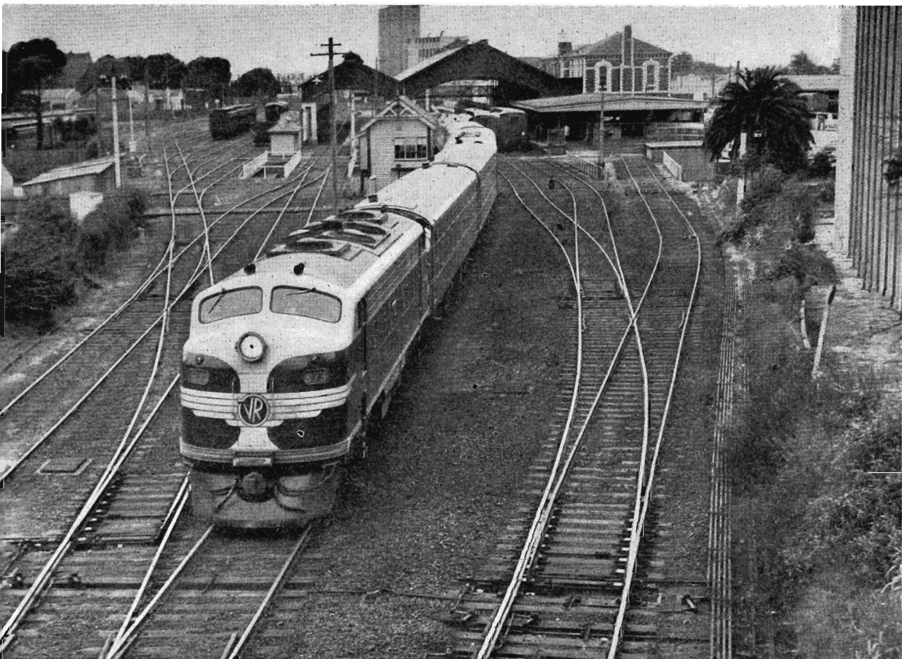
SPECIAL: Typifying Geelong's position as gateway to the Western District, this picture shows a diesel-hauled race train leaving Geelong station en route from Melbourne to Camperdown. The early pioneers' dreams were realized when, in 1890, the railway linked Port Fairy to Geelong.
