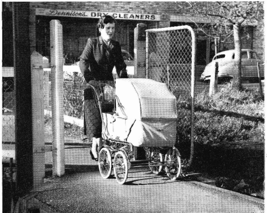
New type pedestrian gates at Poath Road, Hughesdale, make it easy for mothers with prams. The gates normally remain open, and are closed mechanically by the gatekeeper for the passage of trains.
