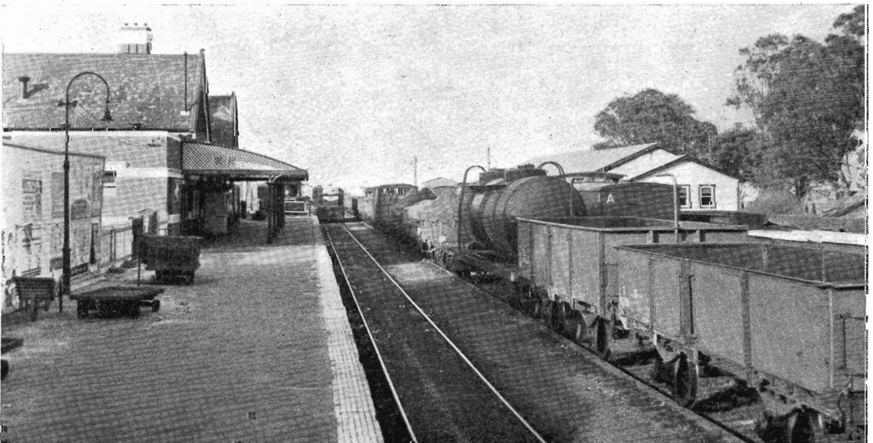
Bairnsdale station yard always presents a busy scene with shunting and marshalling of trains.
