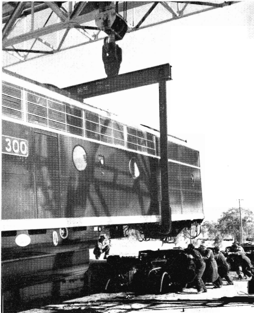
Pushing a 5 ft. 3 in. bogie into position.
