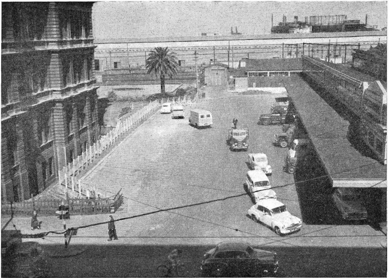
The widened Spencer Street Outward Parcels yard.
