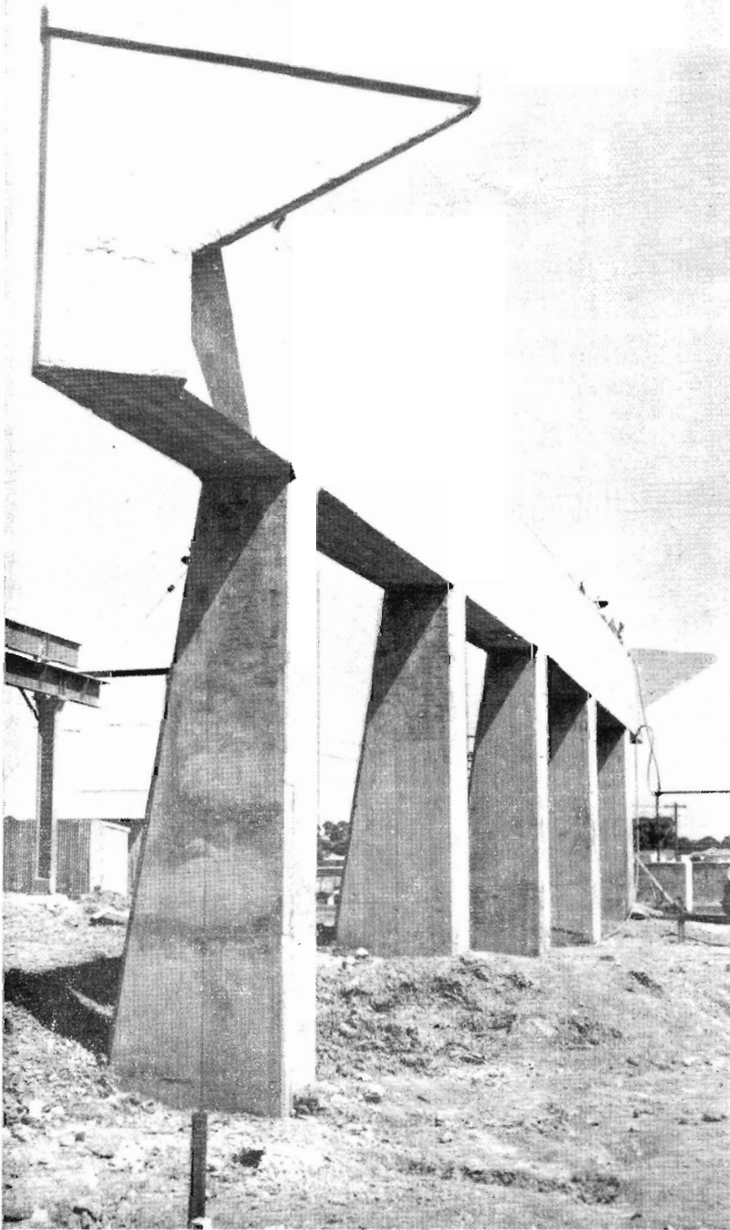
GRADE SEPARATION: At left is a buried pier road bridge at Frankston Road, Dandenong, to crossing. Girders will rest on a ledge on the inside the roadway will be built up on the right. Pier filling for the roadway, hence the name given to. Above are the spans over the railway track at Hill. This bridge is being built by the Country the level crossing, with gates, which raises 6
