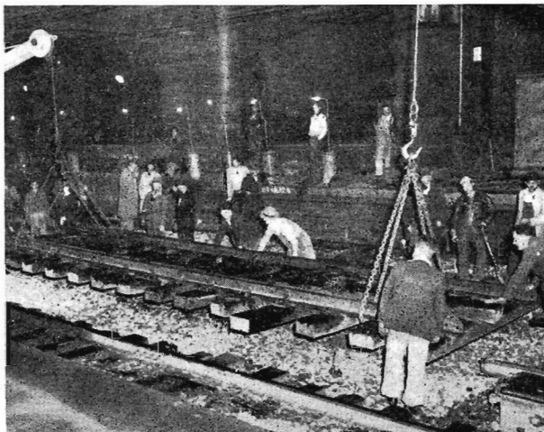
(Left) loading the old trackwork and (right) placing the new trackwork in position.
