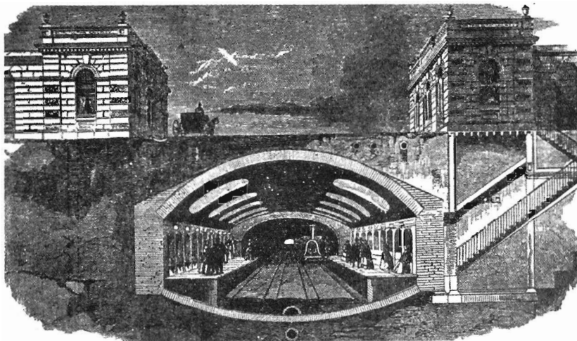
An illustration showing the design for the underground station at Baker Street.
