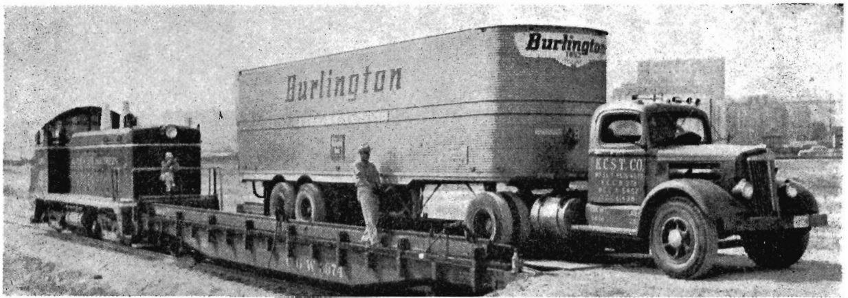
Kansas City Southern Railroad, U.S.A., handles both its own trailers and those of other railroads by "piggyback" service.
