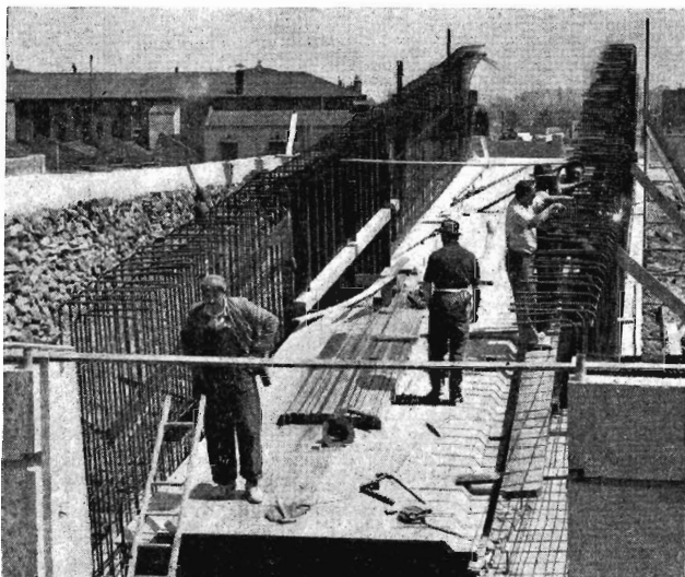
Ramp from main subway under construction and, below, the main subway. Floor level of the subway can be seen by the concrete projection about half-way up the walls.
