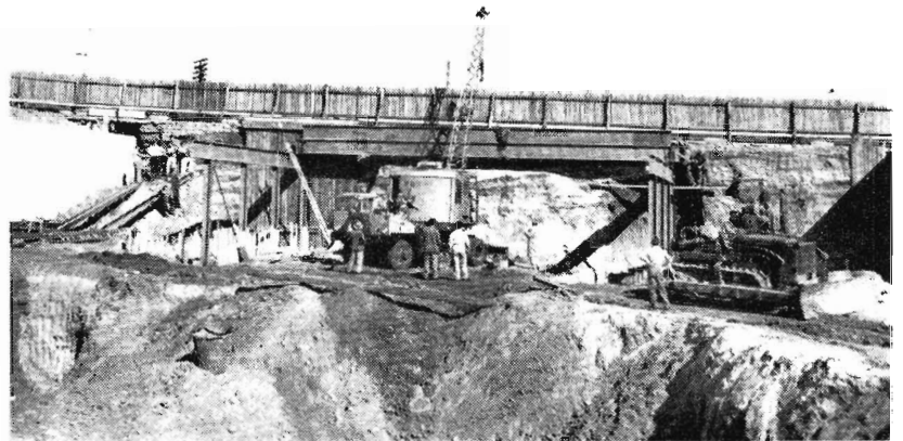
Above is portion of the deck of the flyover bridge for the main line. Low level lines to grain elevators and Corio Quay will pass under this.
