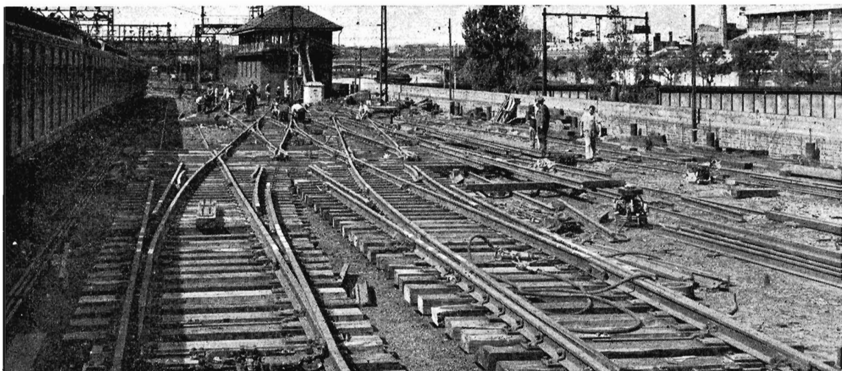
Pre-assembling the points and crossings at the western car sidings.
